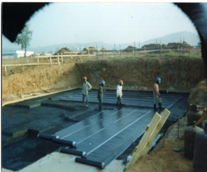
Tanking – Water Retaining
