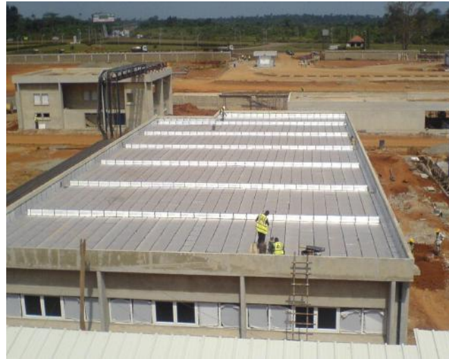
SR / AL Roof Waterproofing
