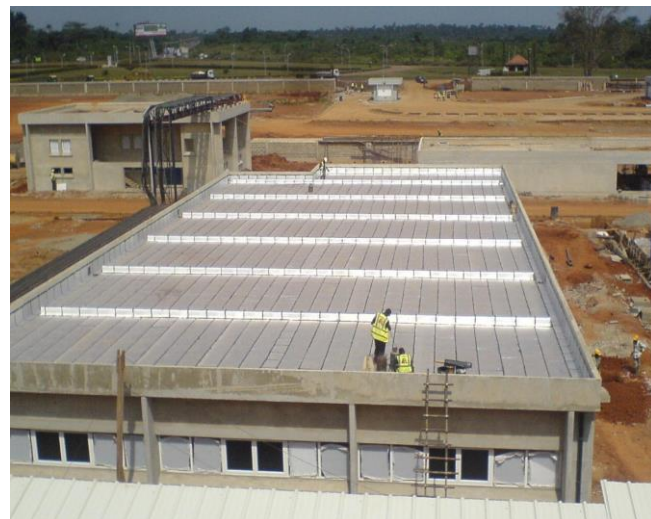
SR / AL Roof Waterproofing
