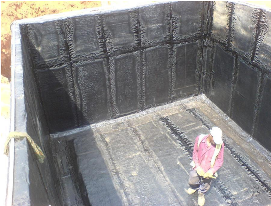
Tanking – Water Retaining
