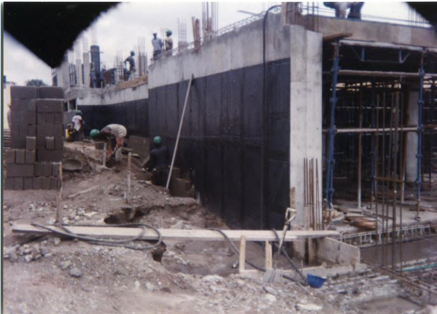
Tanking – Water Excluding
