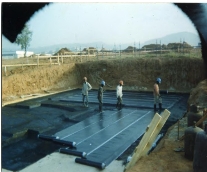
Sub Structure Tanking
