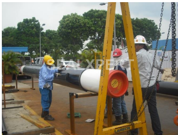
Fig 1: Primer 1027 is applied onto the pipe surface for better adhesion
