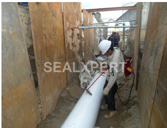
Fig 4: Holiday Test of wrapping before pipeline is buried
